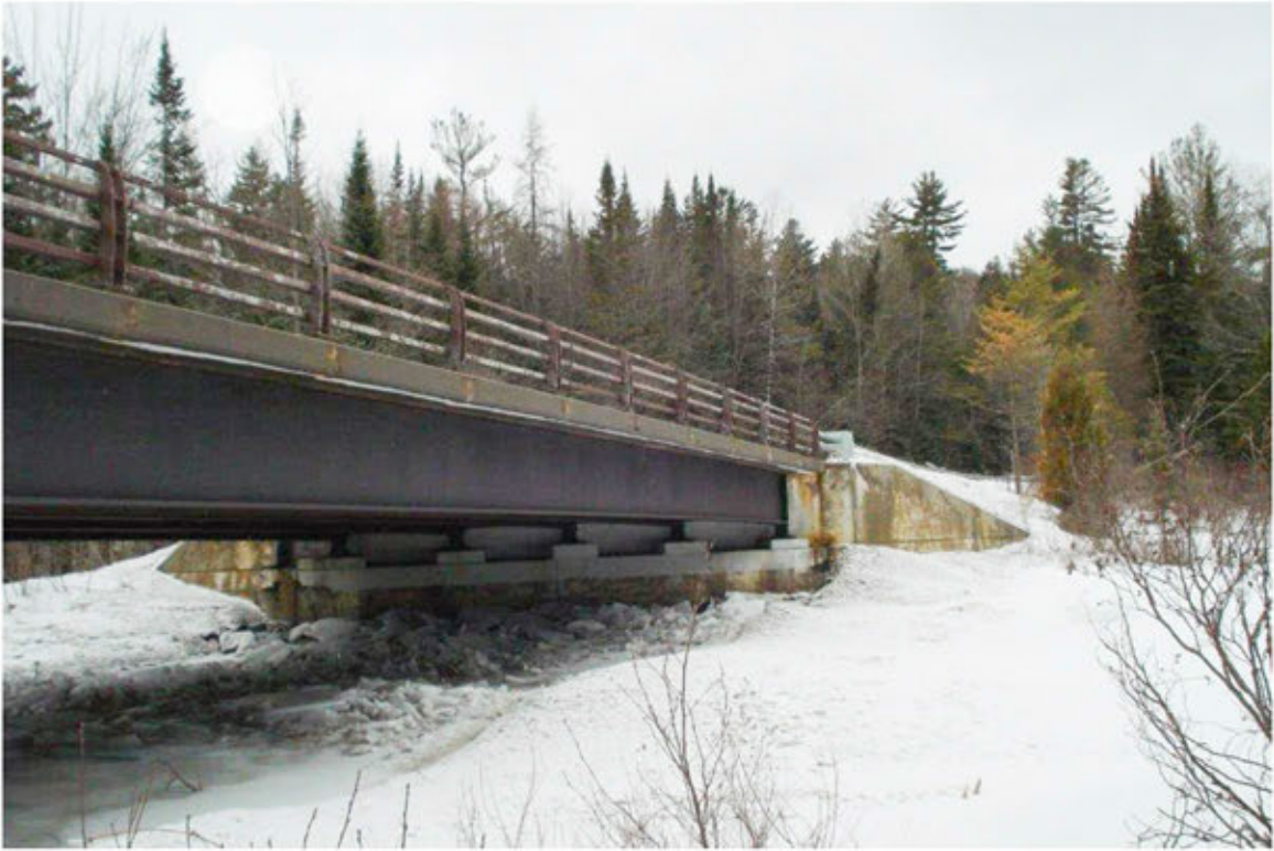
Photo 3 - Route 28N bridge over the Boreas River.
